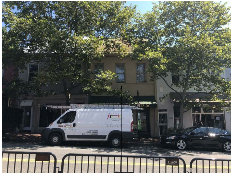
VIEW 1: FROM WISCONSIN AVE NW
